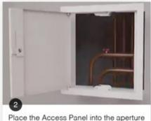
Place the Access Panel into the aperture (no need to remove door or fix supports)
