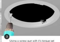
Using a screw gun with it's torque set between 2 and 3, turn the FlipFix screws clockwise until firmly secure.
