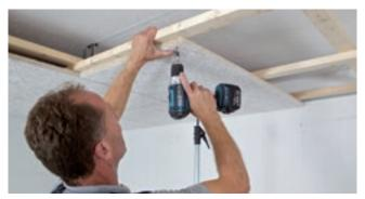
Install the acoustic tiles with the aid of a support. When fixing, press the tile onto the batten using the heel of your hand. There must be no gap between the tile and the wooden batten. For large ceiling areas, begin tile installation from the centre of the room. Observe the installation direction of square tiles!
