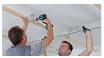
Align the battens using a spirit level or laser level and fix the battens to the hangers, e.g. quick hangers, using 2 screws per side.
