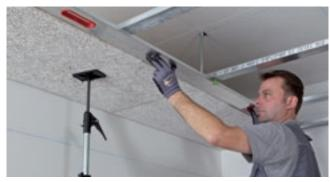
Align the rows of tiles with an installation batten. Tile joints must be positioned centrally under the profiles. No free tile joints are allowed! When installing square tiles, observe the installation direction marked on the back of the tiles.
