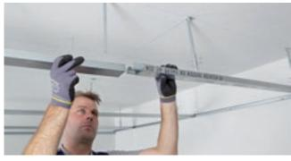
The CD-profile joints should be staggered. An additional hanger at every profile joint.
