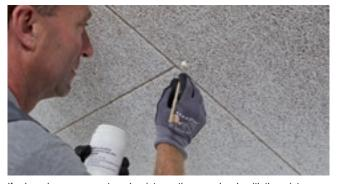
If coloured screws are not used, paint over the screw heads with the paint supplied or a suitable equivalent using a fine brush and suitable amount of paint. Screw heads must be flush with the tile surface.
