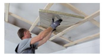
Insert HERADESIGN® acoustic overlays or other acoustic overlays, step-by-step when installing the HERADESIGN® acoustic tiles. Absorber tiles that are pushed between the wooden battens are cut to size.
