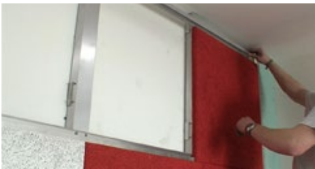
Installation of the upper edge profile. Space required from the ceiling approx. 40 mm. The first tile is moved approx. 10 cm towards the middle, the screws are fixed and then the tile is finally aligned in the grid.
