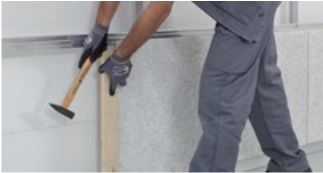
Push the tiles together and align each row horizontally and vertically. Only handle tiles with clean hands.
