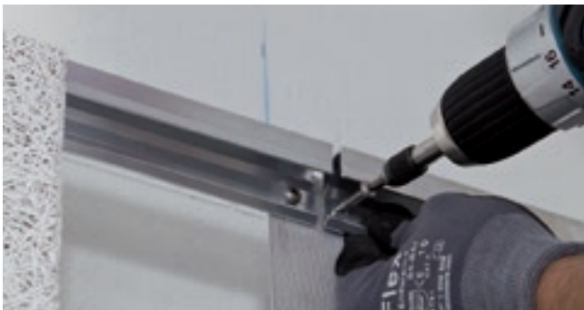
Align the tiles before fixing the perimeter profile with self-drilling screws.
