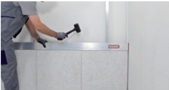
Align the tiles and the main profile before fixing it with the self-drilling screws.
