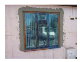
The external corner beads and the mesh of the base trims should also be bedded in. Localised patches of glass fibre mesh should also be bedded over any timber pattresses, pre-coated with R 7.
