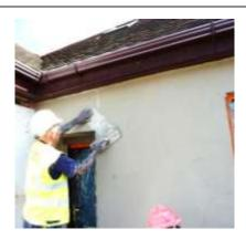
Apply the **Second Pass** of KS HP 14 base coat 2-3mm thick. Rule to line & level removing high points & filling out low points. Allow to semi set & finish the surface with a plastering float or sponge float.
