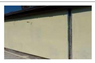
Check the weather forecast to ensure that temperatures will be suitable for application (5°C and rising). The K Systems Silicone TC 15 top coats must be stirred thoroughly before use using a slow speed mixer/ drill & paddle. A small amount of water can be mixed with the product to achieve the best working consistency. Keeping the same ratio of water for all buckets of Sil TC 15 universal for all buckets.
