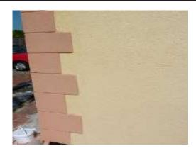
Dash aggregate being applied onto Dash Receiver.
