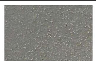
Ensure that the finished surface is flat, as any significant blemishes will not be covered by the thin top coats. The basecoat HP 14 should be given sufficient curing time, moisture free, prior to TC Primer & Sil TC 15 top coat finished
