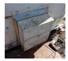
Install aluminium Z spacer supports to either side of gas riser pipes to support louvered powder coated cover plates.
