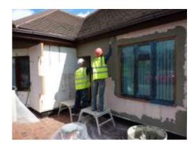
The glass fibre mesh can then be bedded into the first coat of base coat render using a trowel to push the mesh into the render.
