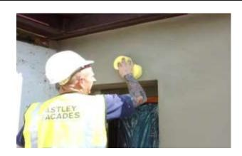
The sponging of the render will leave a lightly textured flat surface with the chips of limestone showing in the surface.
