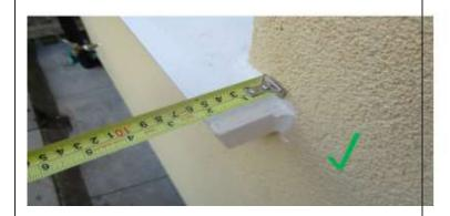
Alu Press Metal capping will be required where the top of insulation board extend beyond soffit or gable wall verges, as system protection & good detailing. Verge Trims should extend 50 / 60mm from all finished render surfaces, to avoid staining.
