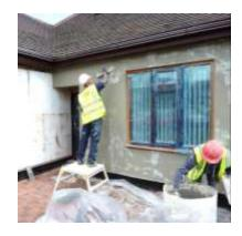
Base coat fully applied at finished depth of 6mm with meshcloth encapsulated and floated up smooth with no surface voids.
