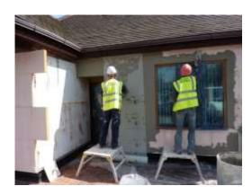
Sheets of the mesh should always be overlapped with a minimum overlap of 100mm. No laps should be placed within 150mm of any reveal or corner.
