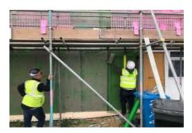
Trim the bottom edge of the glass fibre neatly to marry up with the nosing of the base trim.
