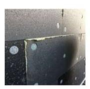
In new build project the insulation board thickness will form the window & door reveals footprint to receiver basecoat render. In retrofit project where the window frames will not be moved, thinner Insulation boards will be adhesively fixed & returned into the frame abutment with compriband seal tape. See package details.
