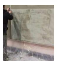
Diagonal stress patches of mesh (approx. 250mm x 350mm) shall be installed to all corners of any reveals as per the standard KS details.
