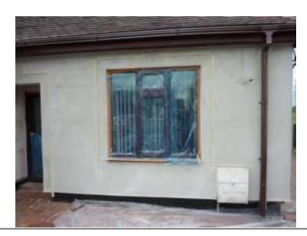
On properties with external rainwater pipes it is beneficial to fit temporary flexible sock pipes or rigid pipes that will guide rainwater away from the face of the building.
