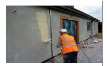
The TC Primer coat should then be allowed to dry for up to 24 hours before the next coat, using Sil TC 15 is applied.
