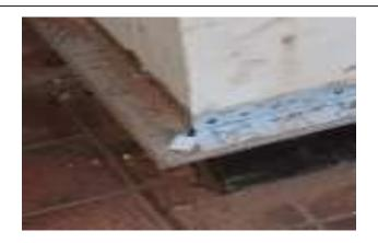
Alternatively if a thick coat render finish such a dash aggregate, scratch texture coat or brick effect render is to be used then a more heavy duty base trim as shown may be specified.
